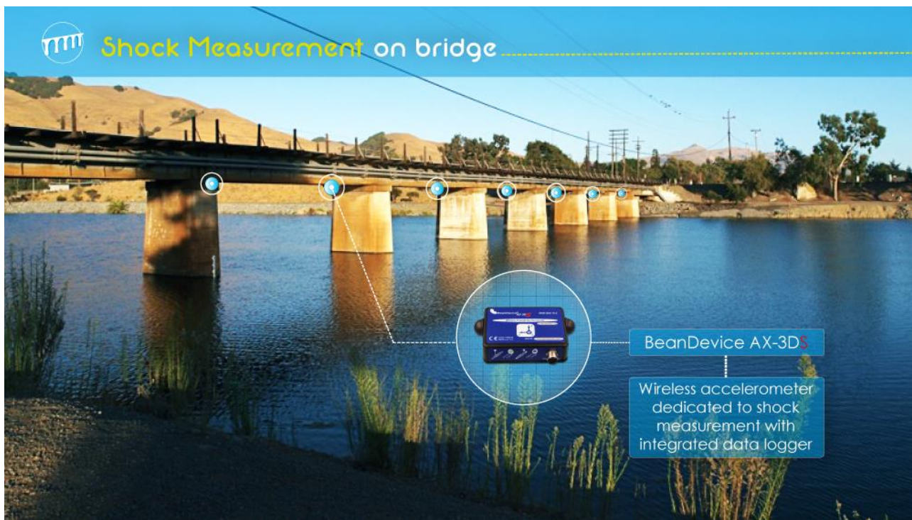
Figure 4: Sinking, Shock and Crack detection on Bridge
