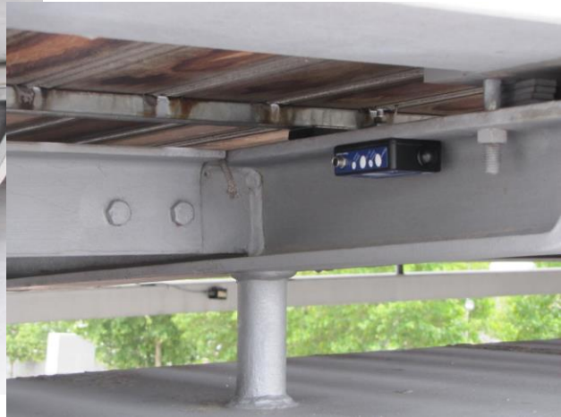
Tilt Measurement on bridge ( max measurement range +/-1,5°)
