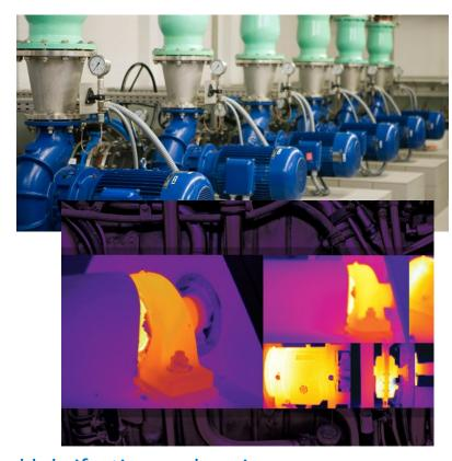
A bad lubrifaction on bearings can lead to temperature increase
